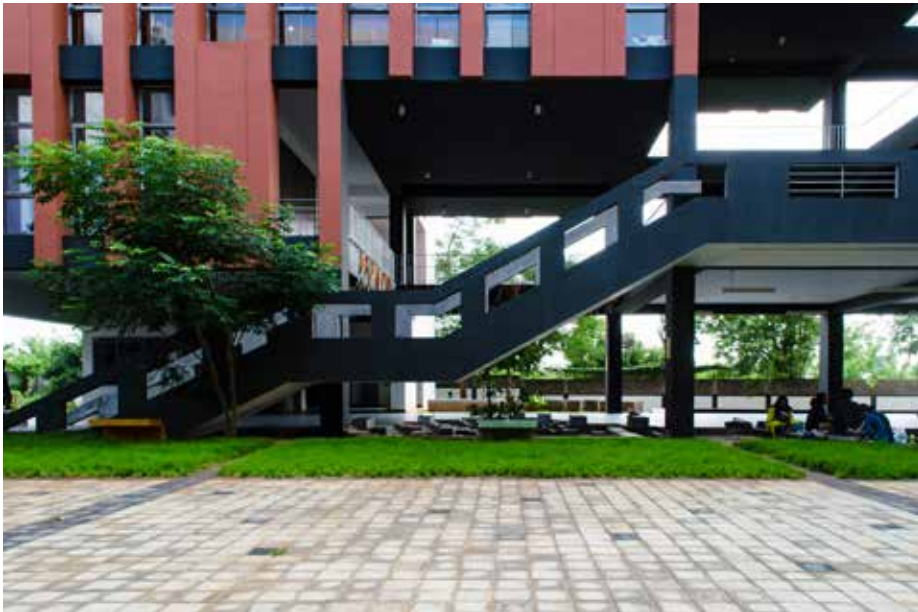
Entrance staircase tying the ground plane to the upper courtyard
