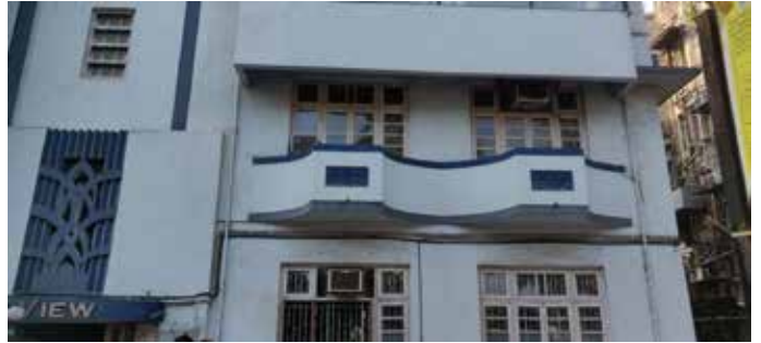
Curvilinear balconies of Art deco buildings at Oval Maidan with tropical details in RCC
