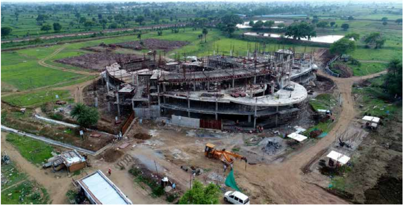
Under Costruction View
