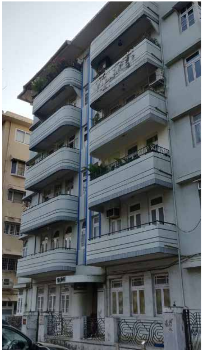
The Fairlawn building which overlooks the Oval Maidan, distinguished by the style of its balconies and compound wall.
