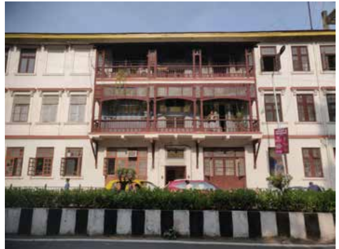
Concrete balconies replaced timber but followed the same design pattern. The role of the carpenter was replaced by the mason in the new designs
