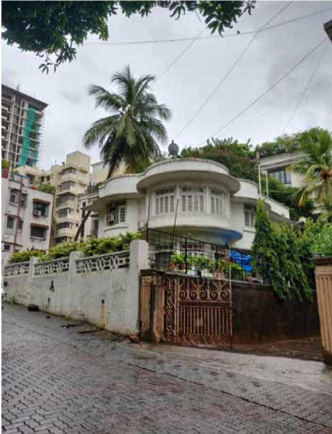
The chajjas of the Art Deco building, also called 'eyebrows', protect the building from harsh monsoon rains
