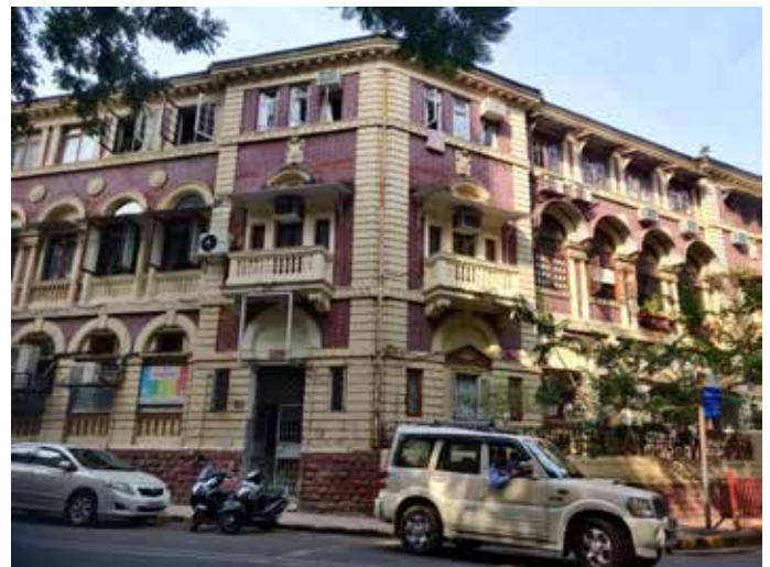
Experimentation in the chajjas of buildings which cuts direct sunlight and enhances the aesthetics of the building
