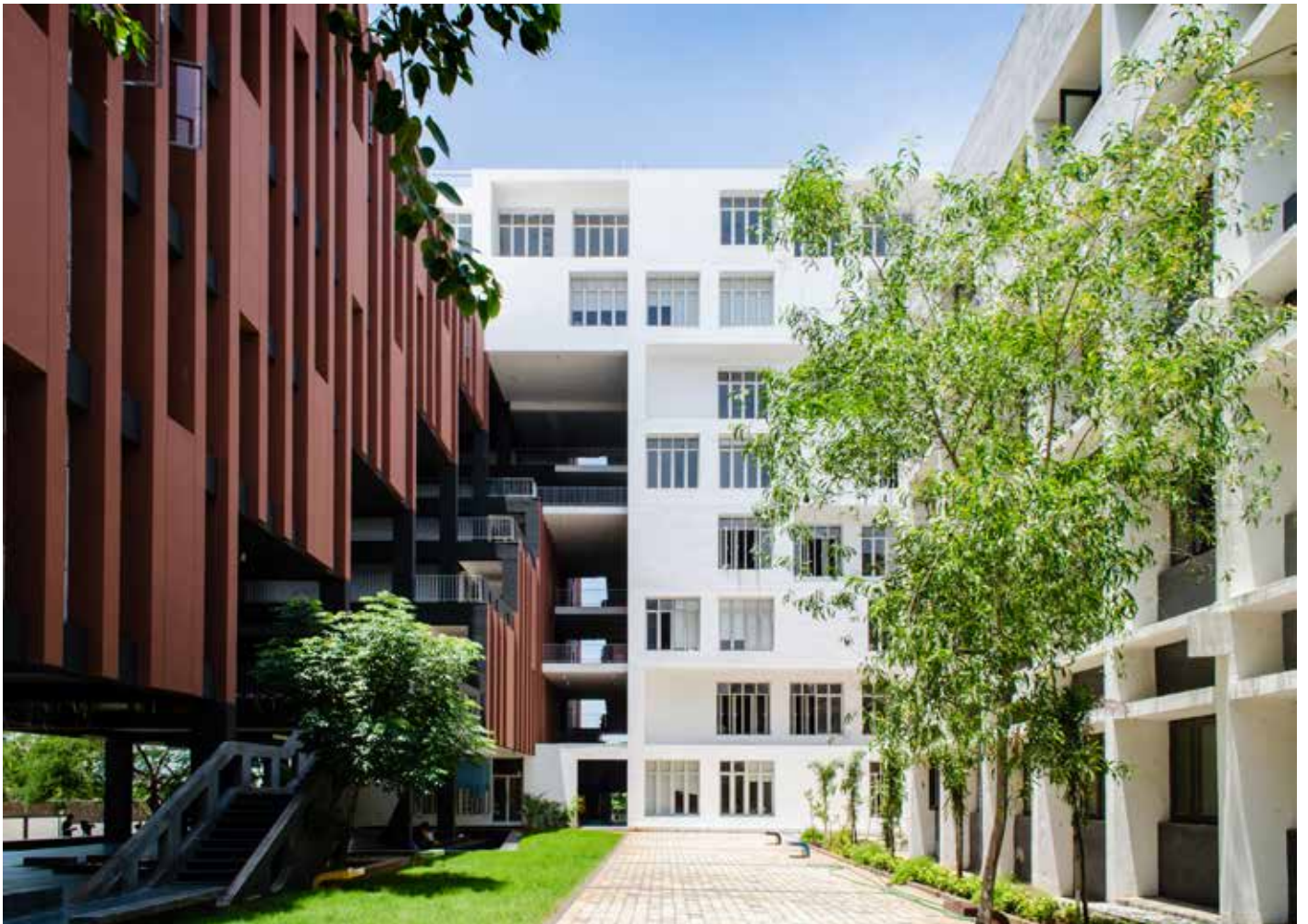
A view of the sectional courtyard, tying the building to the ground plane
