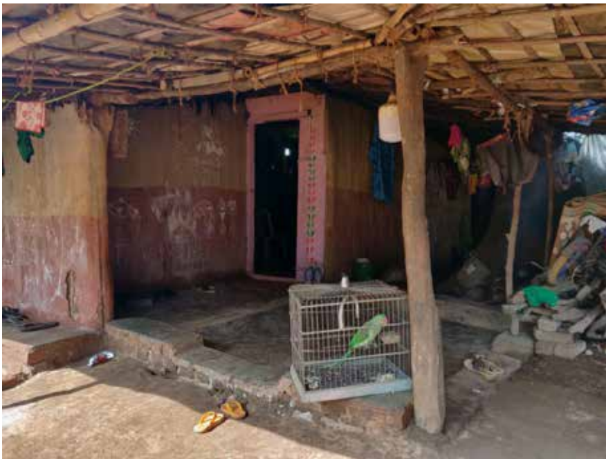
House of the Warli tribe, with an offset entry made by cob walls which helps maintain the temperature of interiors.
