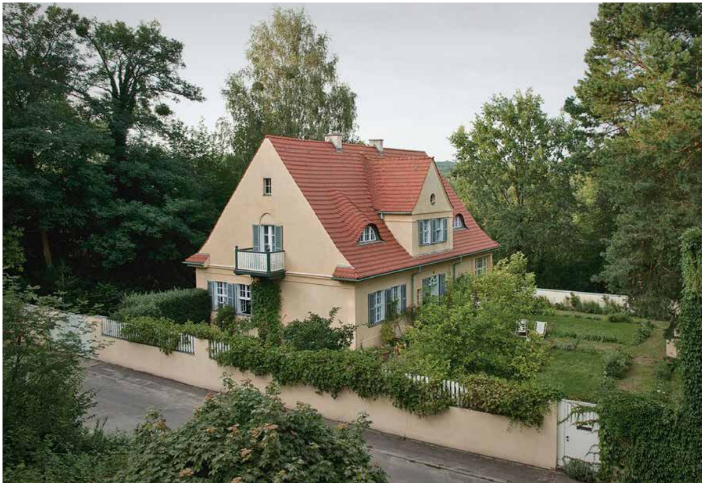
Mies uses the elements in the roof like the central gable dormer window, eyebrow dormer windows flanking either sides and minimal ornamentation to highlight his building (Source: https://ofhouses.com/post/146589627148/322-ludwig-mies-van-der-rohe-riehl-house )
