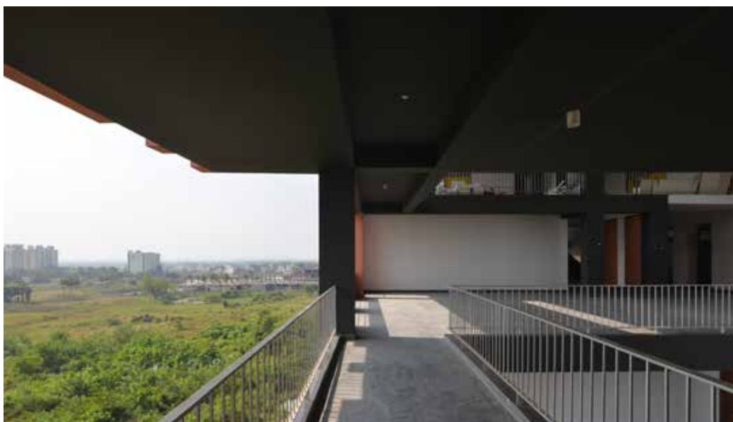
Views to the reserved forest, as seen from the courtyards.
