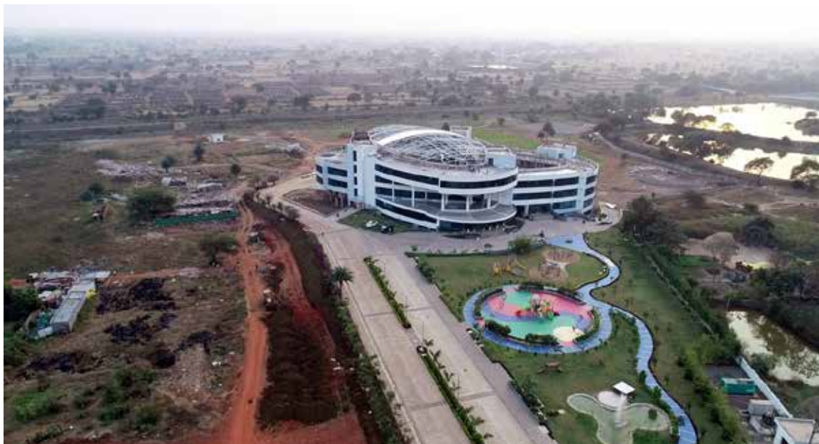
Site Aerial View
