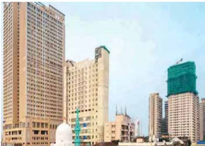
The newer post-modern buildings with 'dead' facades and sometimes no scope for cross ventilation and protection from rain
