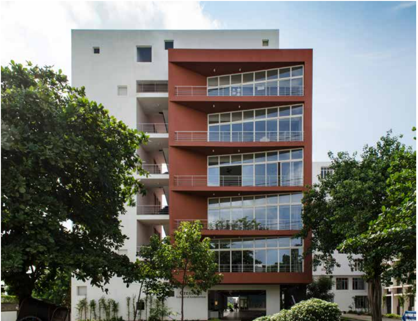
Front elevation and main entrance into the building
