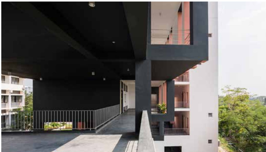
Open breezy nature of the courtyards, offering views to the surroundings while tying the building together
