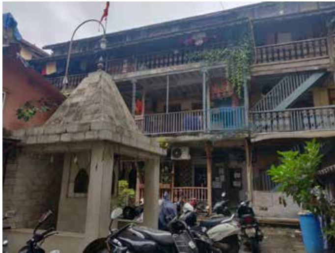
Well- ventilated corridors in front of houses in the chawls which cut off direct sunlight and allowed people to interact
